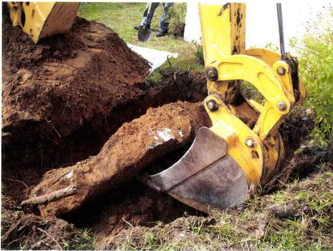
Picture 2: UST 1331Albatross concrete removal in progress. UST located under concrete.
